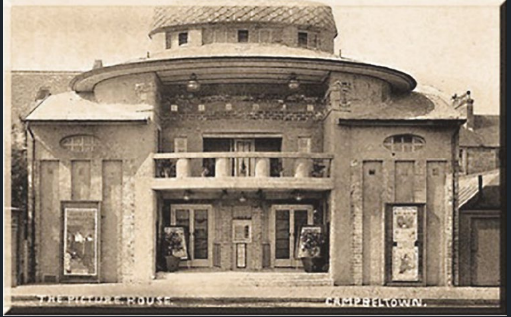
fig. 1. Frontage to Hall Street, 1913
