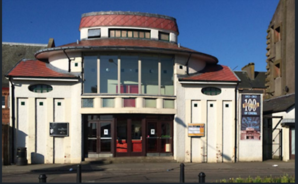
fig. 3. Frontage to Hall Street, prior to conservation Photo: Ron Inglis
